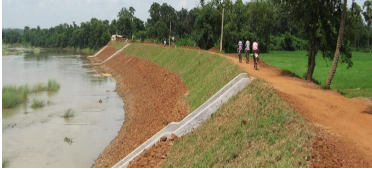
Figure 4- River plain with embankments
